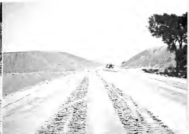
Cut slopes with transition at the ends of cuts and protected with top soil present a natural appearance
